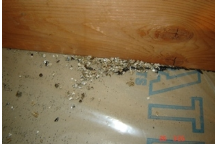
Figure 2. Vermiculite in attic
